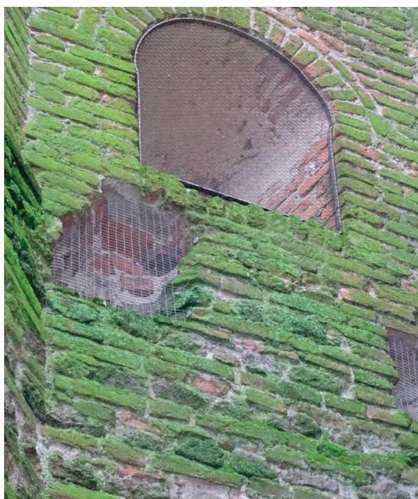
Photo 23. Algae colonies on a moist ceramic brick wall.
