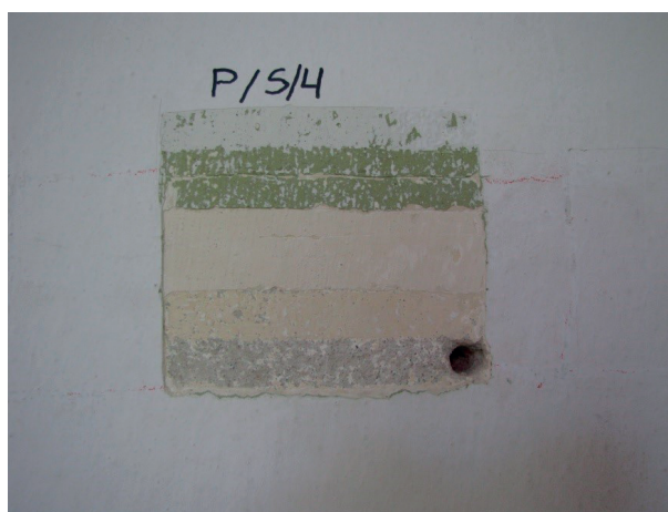
Photo 22. Stepped probe showing the arrangement of layers of plasters and paintings on the wall.
