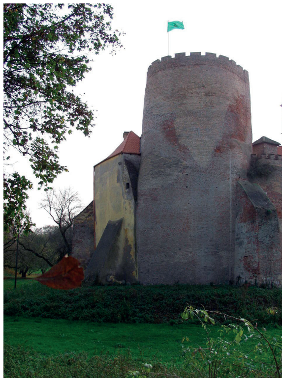
Picture 10. The present state of the tower: the “stains” on top of the walls indicate the restored parts of the tower as well as areas with increased amounts of moisture in the walls
