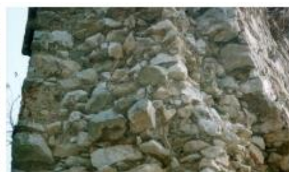
Image 100: building work of the opus emplecton type, clearly visible before the reconstruction: thick wall is made of three layers. First, two parallel walls were erected and the space between them was filled with stones and crushed rocks, quicklime was added and cooled with water - thus the filling changed into a monolithic conglomerate core which is however only poorly linked with stones in circumferential walls, which fall off.
