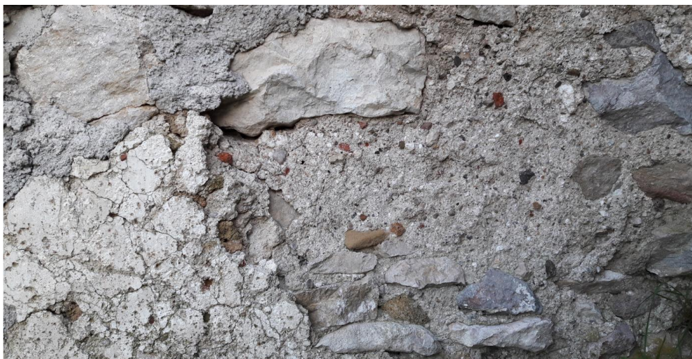
Crushed bricks in the castle walls mor- tar.
