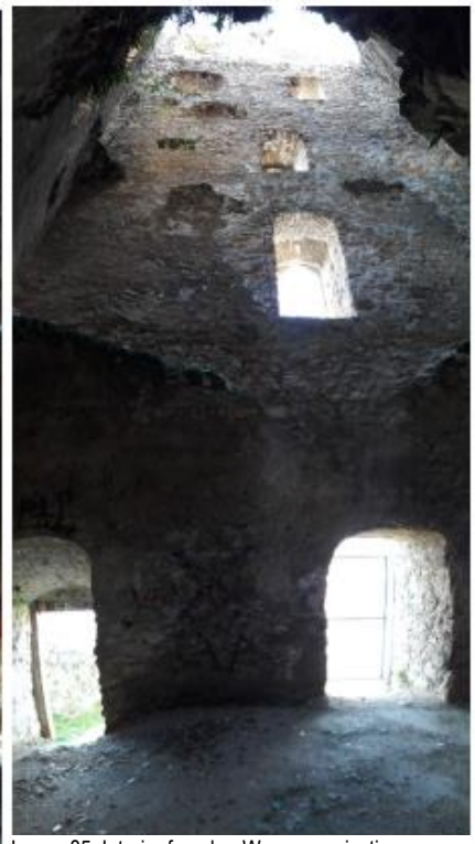
Image 85: Interior facade - W: communications were directed to the interior court yard. Two top windows are equipped with sedilias.
